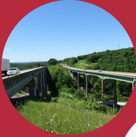
Canoe Creek Bridge
