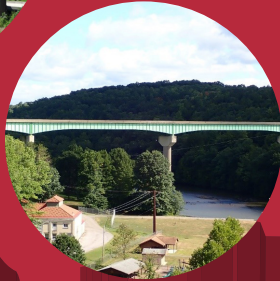
North Fork Bridge
